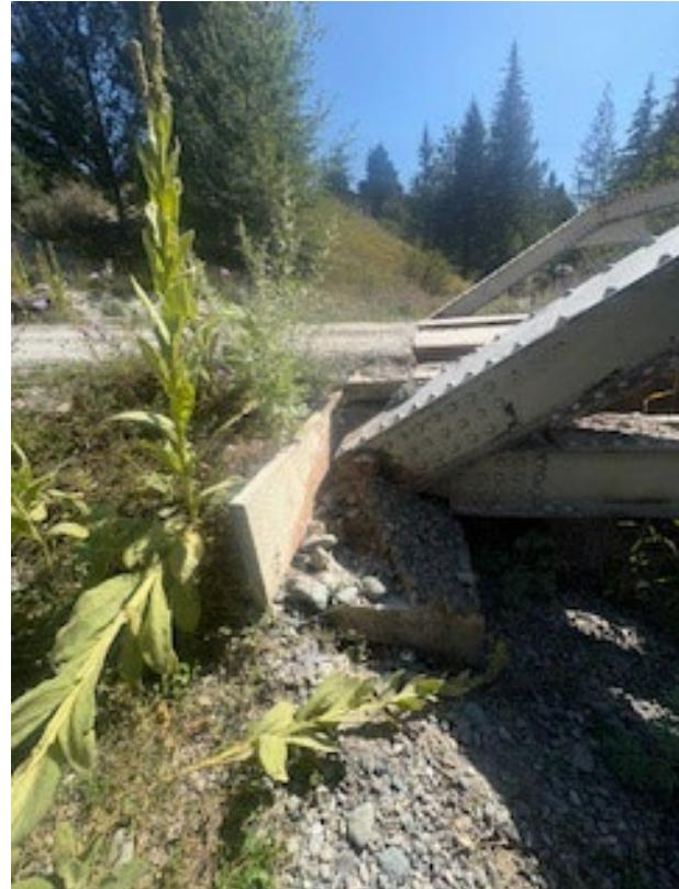
The only nearby structure is the bridge we want to repair. The bridge was put in place in 2000. Its main steel structure is in good condition; it is only the wood decking that is rotting due to age and natural deterioration.
